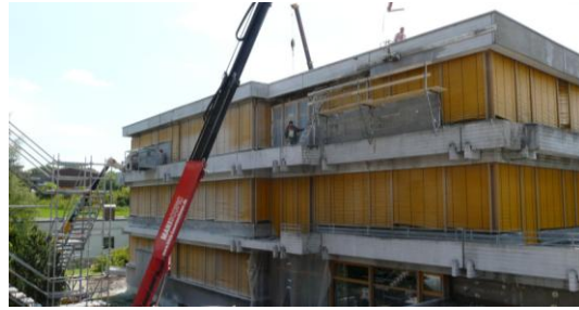
Fig.8 Realschule Buchloe, removal of precast concrete façade
