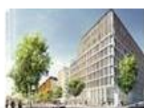
Green Link Office - Lyon
