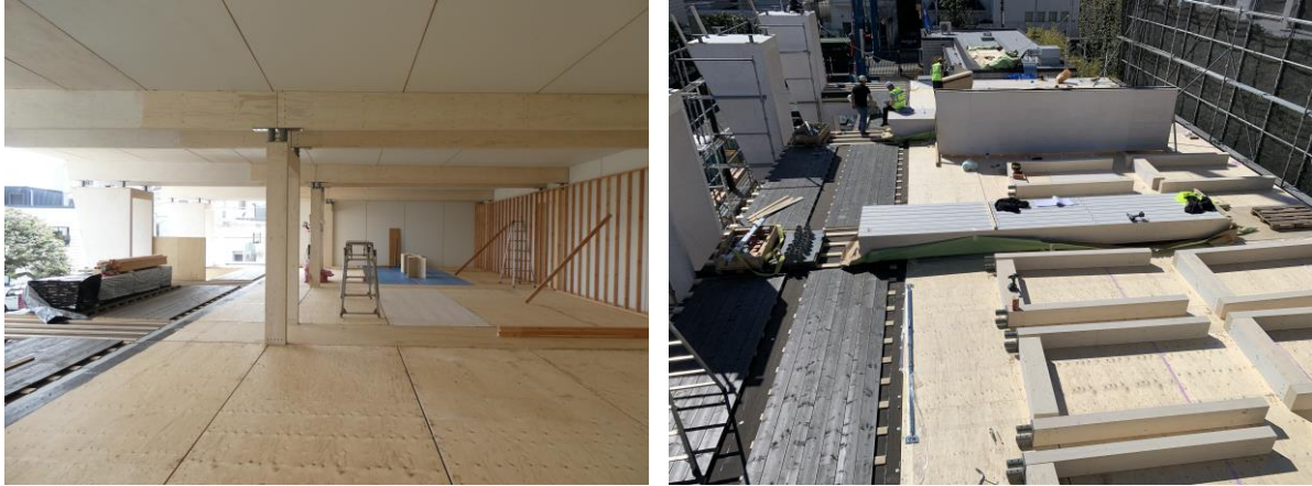
Image: Wooden elements make the building quick and easy to assemble. The pavilion was built in Finland and assembled in less than two weeks in Japan.
