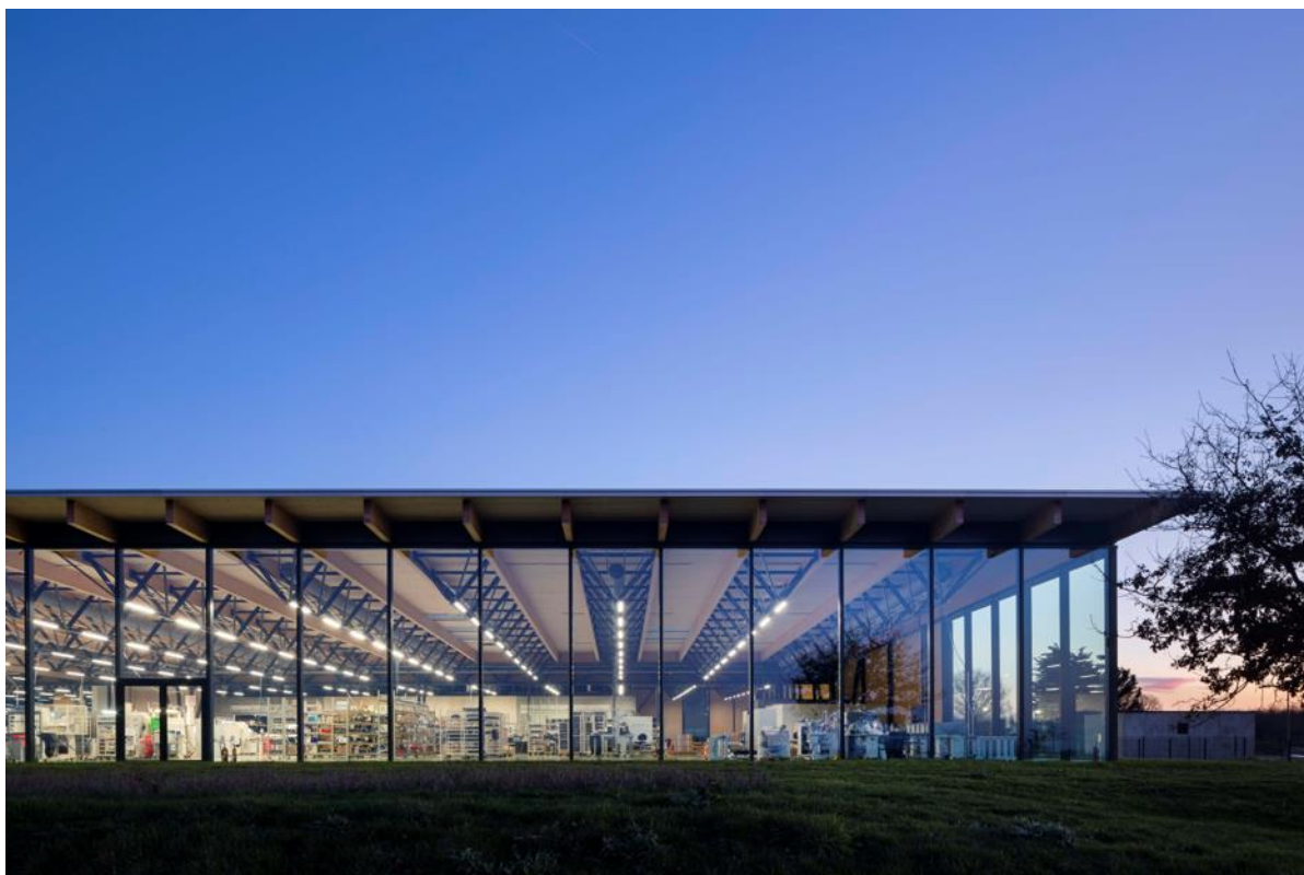
Figure 1 : Façade Nord ©H. Abbadie
