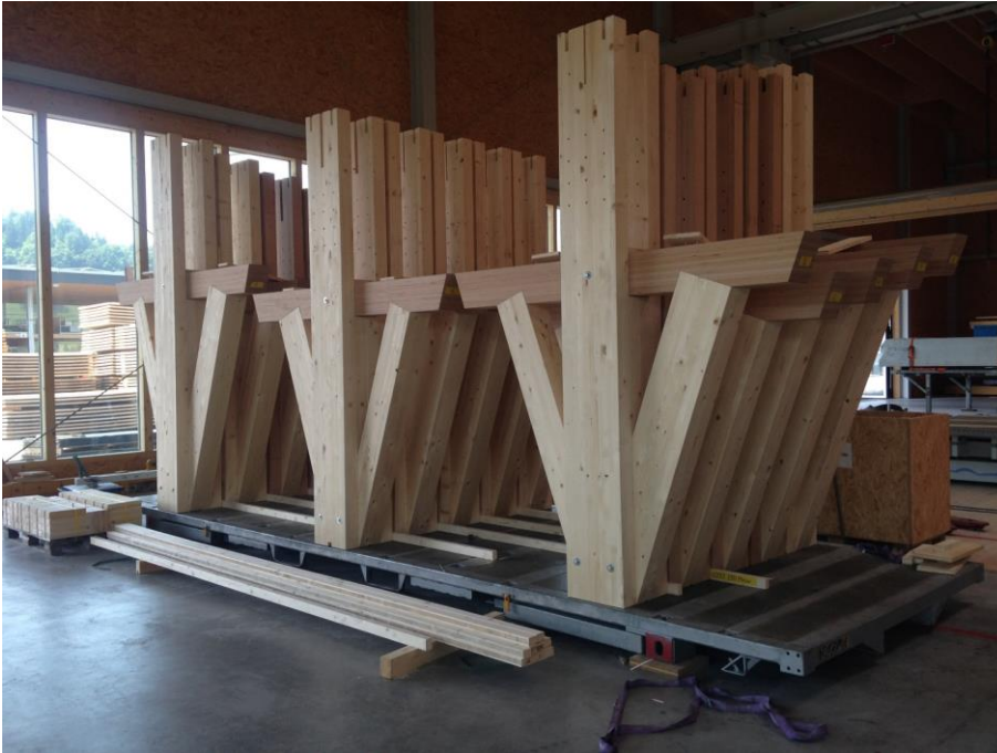
Figure 5: The V-form pillars with the BauBuche floor and lateral consolidation poles for absorption of the loads from the storeys above were assembled in the factory. The varying strut dimensions result from the different forces in the boundary elements; the different heights are due to the pitch of the carriageway aisle.
