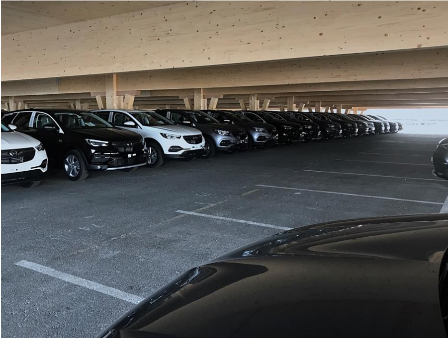
Figure 13: Parking situation during construction phase on ground floor
