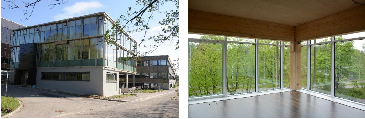
Figure 9: ETH „House of Natural Resources. Building from the outside (left) and office with post-tensioned timber frame (right)
